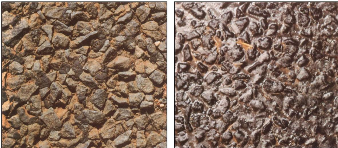
*Figure 20: Hungry coarse seal coat before (left) and after applying a surface enrichment of 0.7 L/m<sup>2</sup> of cutback bitumen (100-0-20)*
