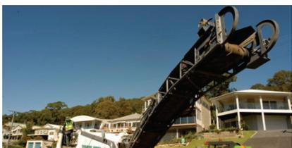
A profiling machine removes the wearing (top) course from a flexible pavement, ready for a new surface to be applied and the removed material to be returned to an asphalt plant for re use.
